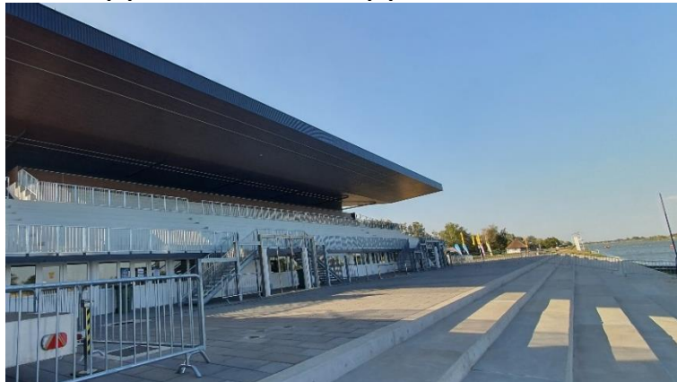
Picture of a Grandstand
